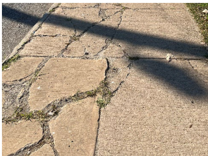
Existing Sidewalk Condition:
