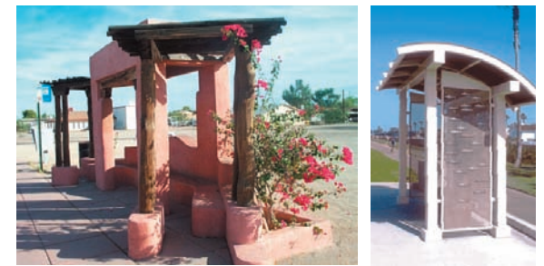
Custom designed shelters in Arizona and California that relate to the colors and materials of local architecture
