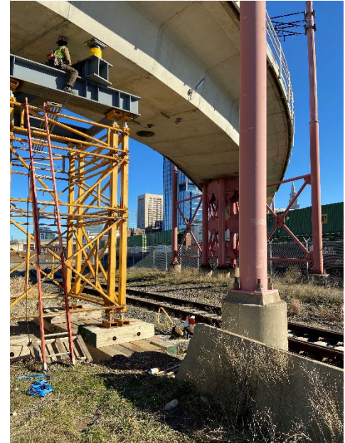
Figure 47: Jacking Process on the Waterfront Line Bridge
