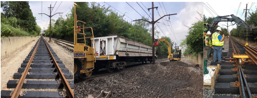
Figure 61: Light Rail Ongoing Track Rehab
