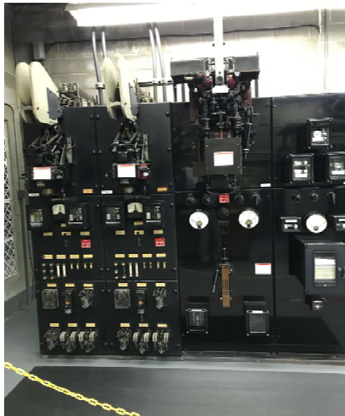
Existing 600 VDC Switchgear
