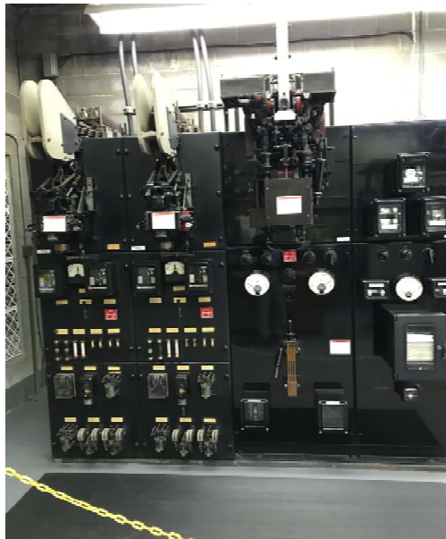
Existing 600 VDC Switchgear
