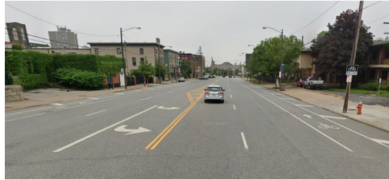
W. 25 th Street looking northbound towards Detroit Avenue
