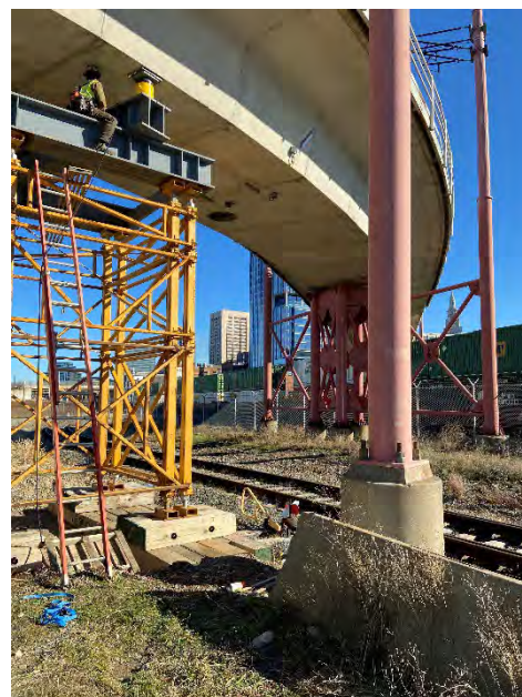
Figure 49: Jacking Process on the Waterfront Line Bridge
