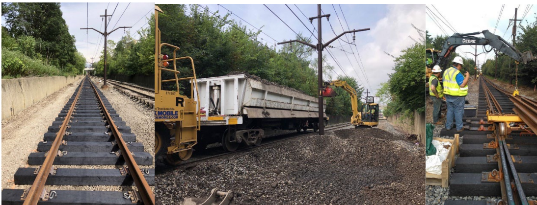
Figure 62: Light Rail Ongoing Track Rehab
