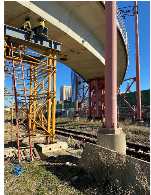
Figure 49: Jacking Process on the Waterfront Line Bridge
