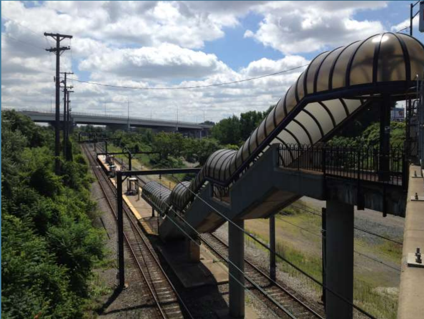
Existing Condition – View of Station from Bridge
