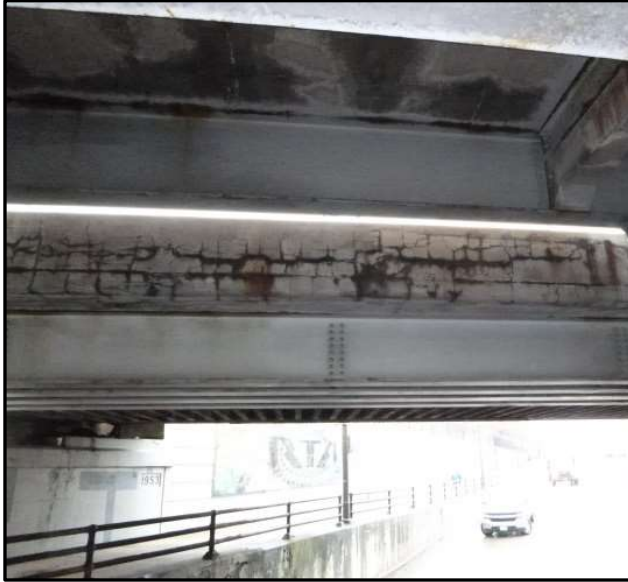
Concrete Deck on Steel Beams
