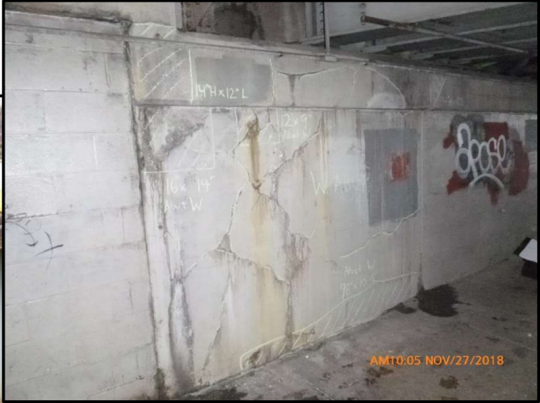
Concrete Foundation @ Ends
