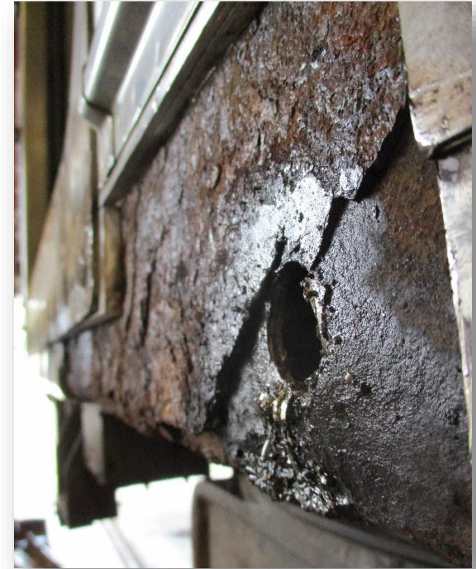
Corrosion Section Loss
