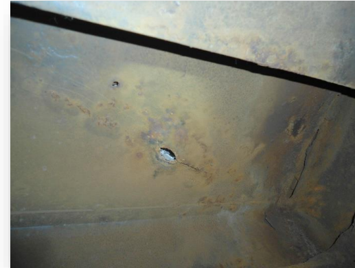
Corrosion Hole/Crack in Articulated Structure
