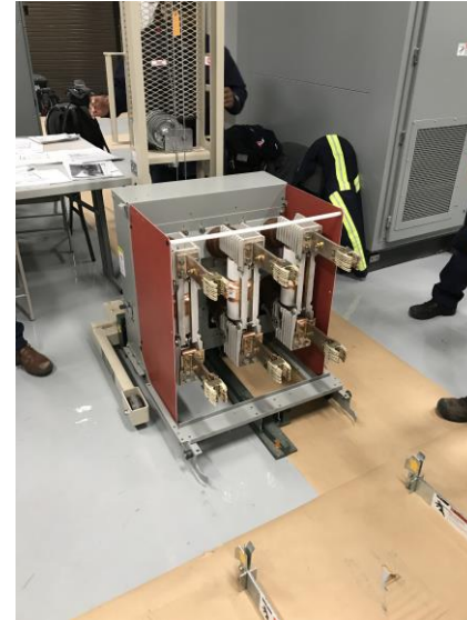
Installing new equipment
