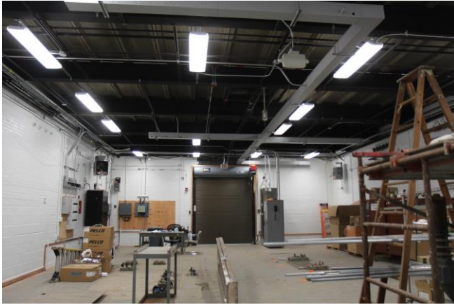
West 65 th Street Station following removal of old equipment
