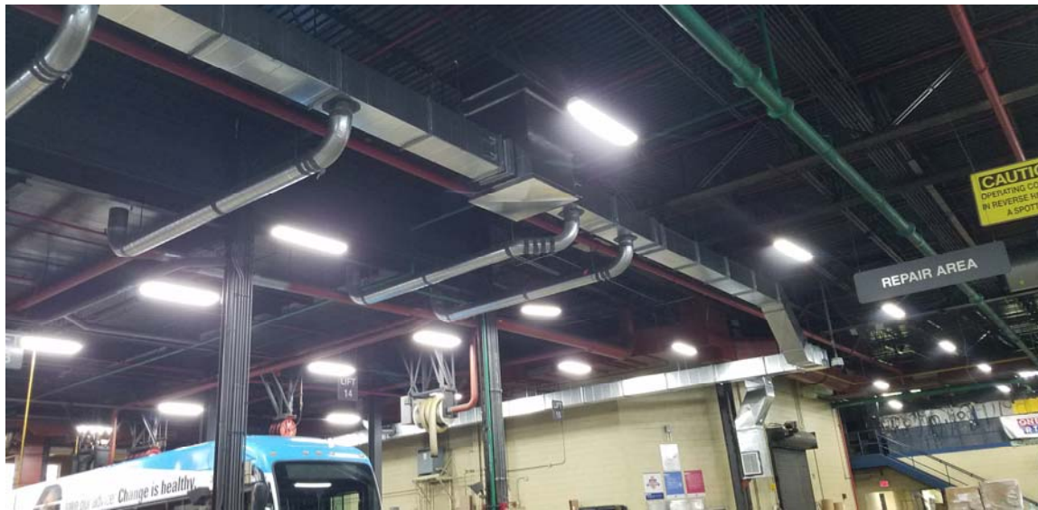
New Ductwork
