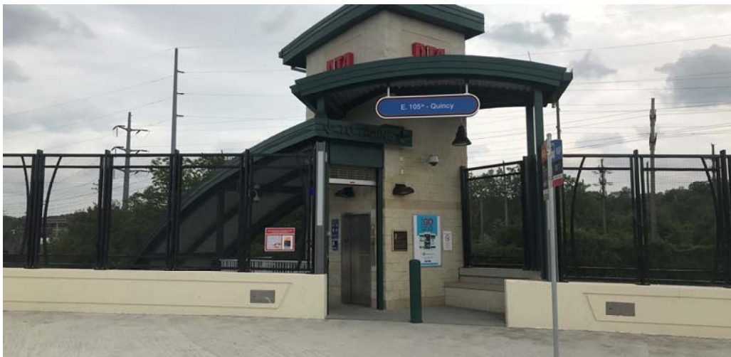
E. 105/Quincy Redline Station Construction $4.0M
