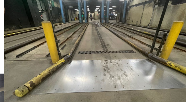
Bus Wash Entry Lane
