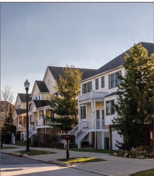
Townhouses at Mill Creek
