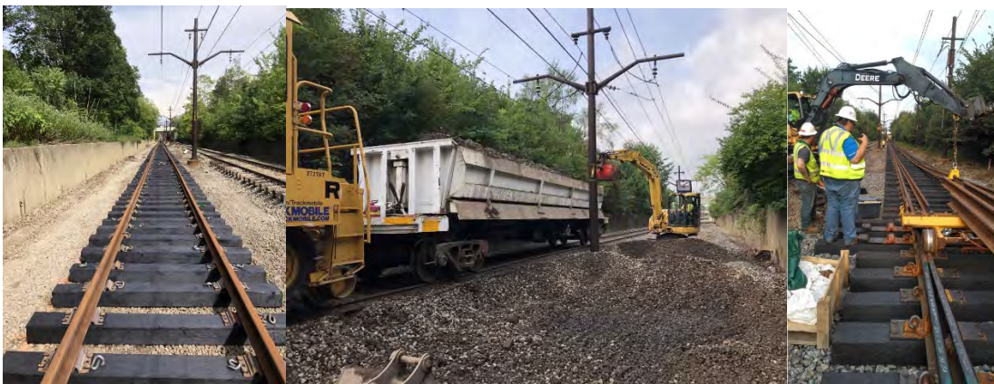
Figure 62: Light Rail Ongoing Track Rehab
