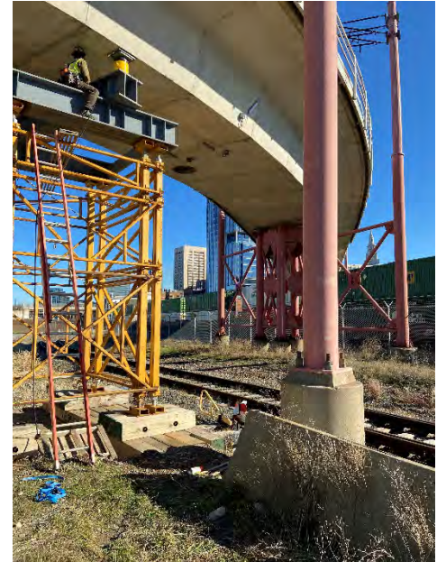
Figure 45: Jacking Process on the Waterfront Line Bridge
